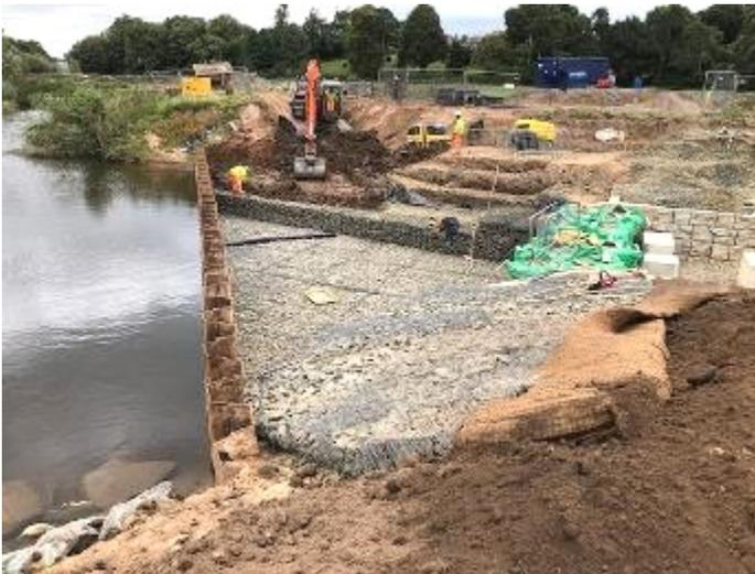
The Bevere fish pass is unique in its design. A regular fish pass takes the form of a 'ladder' with each rung stepping up a level. In contrast, the channel at Bevere is a long, gently sloping course with blocks cast into the base of the channel to break the water flow and create conditions where fish can swim upstream comfortably for the first time in over 170 years.
