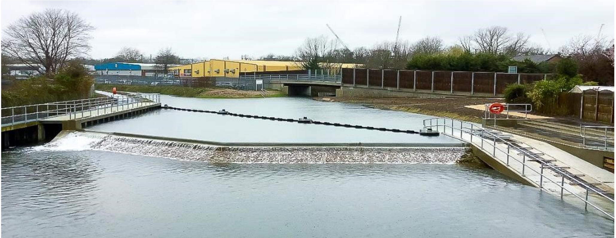
Greenford was responsible for the construction of a weir alongside a fish and eel pass at Green Lane as part of the Maidenhead Waterways project.
