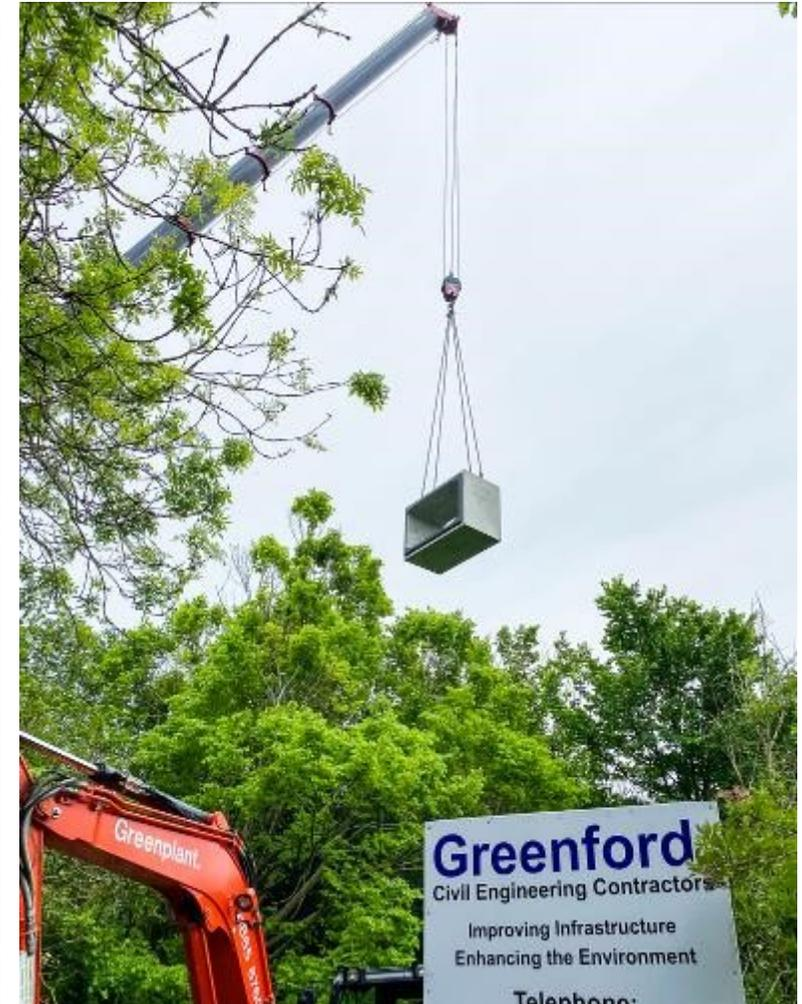
This project involved the clearing of an overgrown culvert at a historically protected farm in Witney. Greenford created and installed a strong culvert structure to allow water to continue to flow effortlessly under the bridge.
