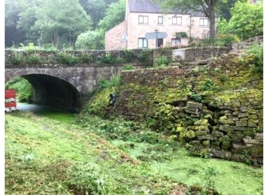
Greenford carried out the work on this historical flood gate system built in the canal walls and bed. The remains were discovered during the initial excavation which Greenford rebuilt and replicated in order to form the new wall.
